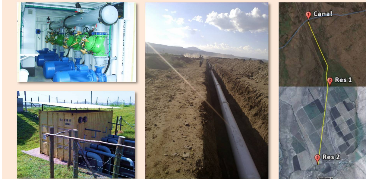
2017 Dejenja chemicals project in Ethiopia - 700 ha of undeveloped land - 4.8 km distance from Irrigation canal to the seconded reservoir -70m difference in ground level
