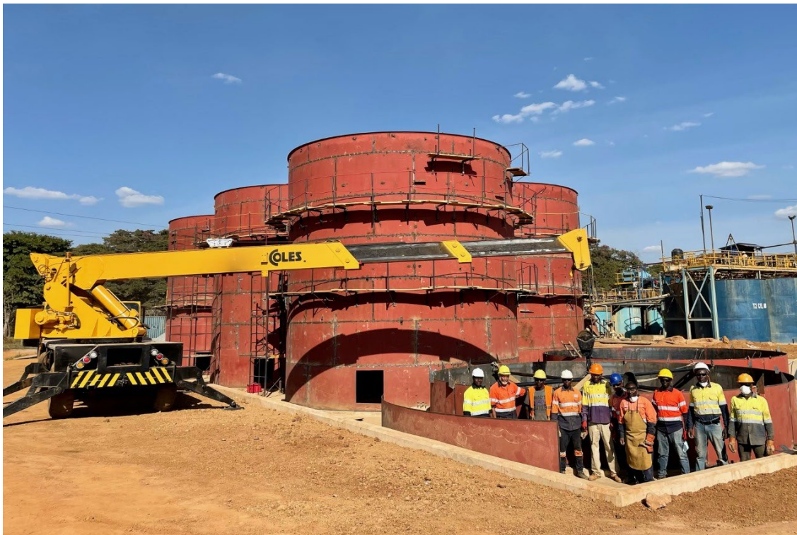
Figure 3: CIL Tank Construction at 1,000 tpd Plant at Buckreef Gold Mine (July 2022)
