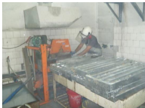
Core Cutting in Progress
