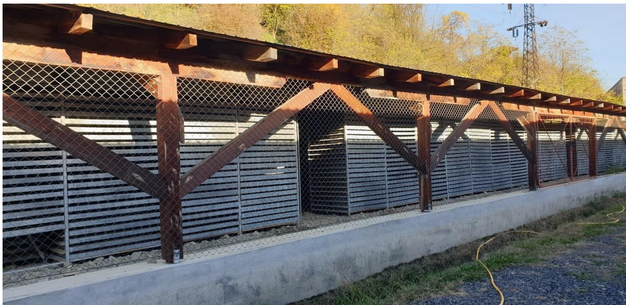
Figure 10.3: Permanent Core Storage Facility
