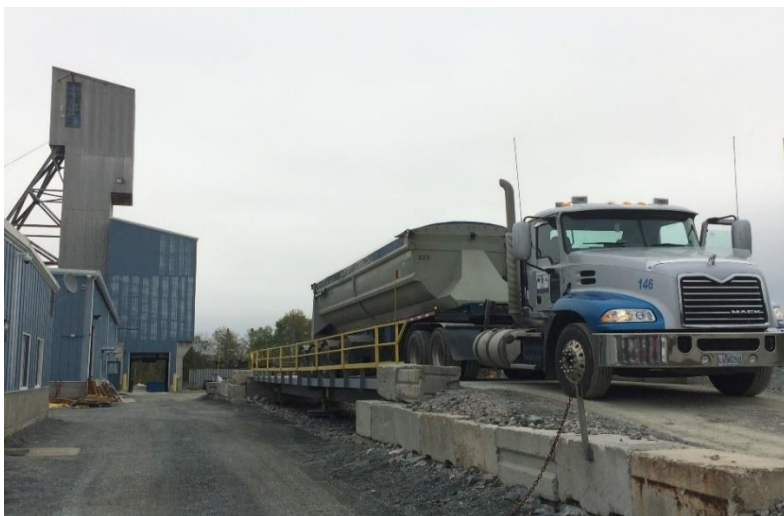
Truck scale and shaft headframe
