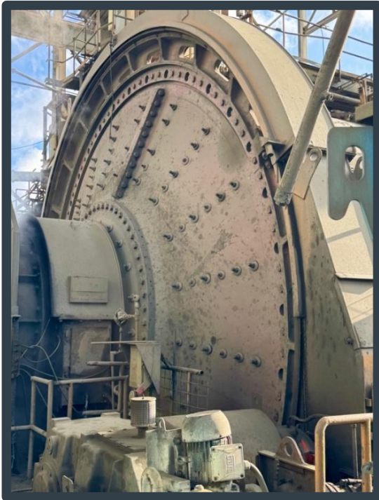
Sag mill at the Campo Morado plant
