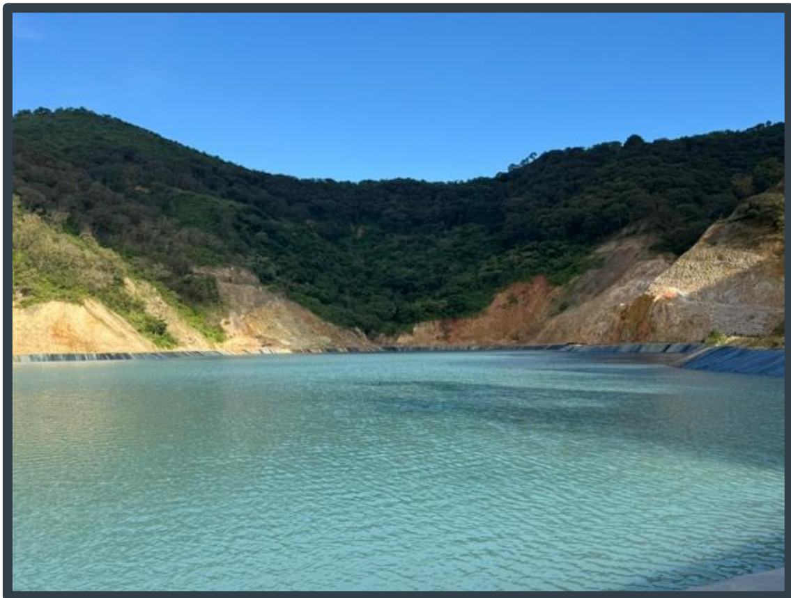
Tailings storage facility at Campo Morado
