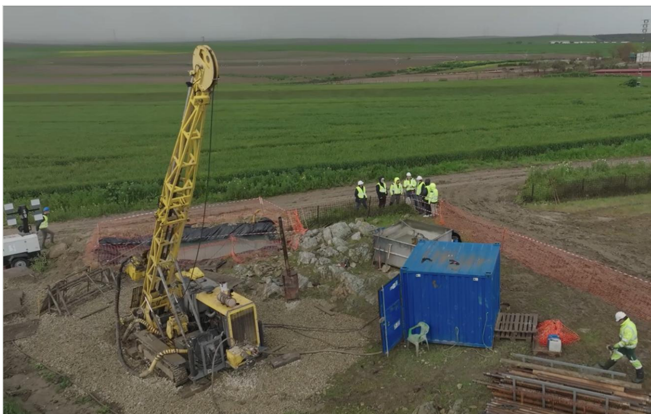
Figure 10-1 Photograph of Diamond Drilling in Progress at La Romana
