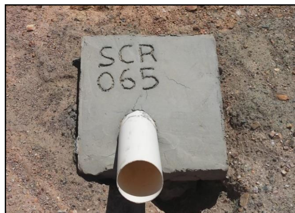
Figure 10-2: SRC-65 Cemented Drill Hole
