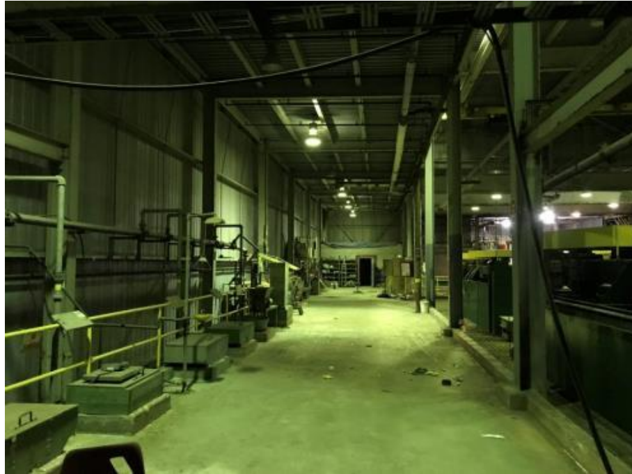
Figure 18-45: Large Main Deck Maintenance Bay
