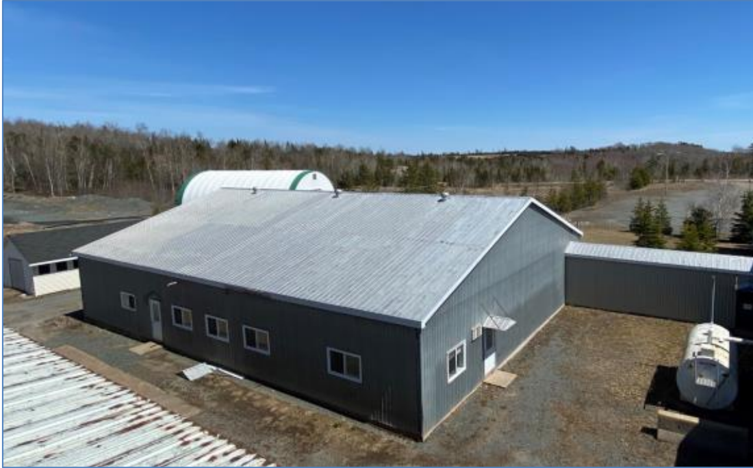
Figure 18-15: Mine Technical Services & Operations Building
