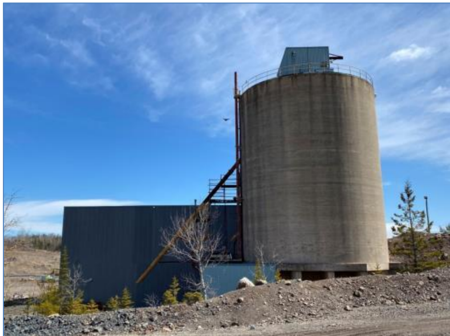
Figure 18-33: Existing Mill Fine-Ore-Bin (Silo)
