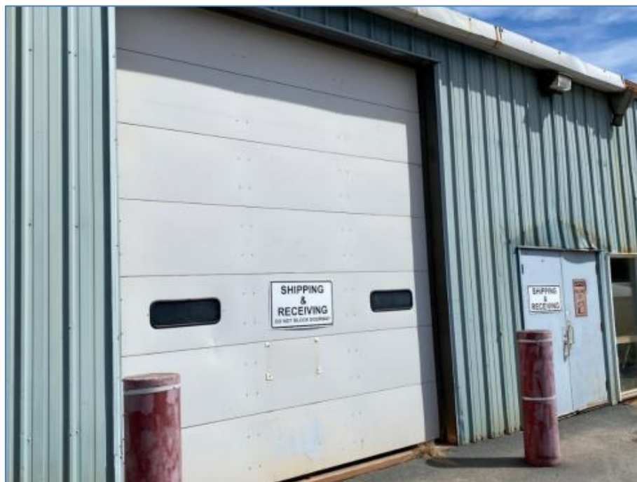
Figure 18-17: Site Warehouse Receiving Bay
