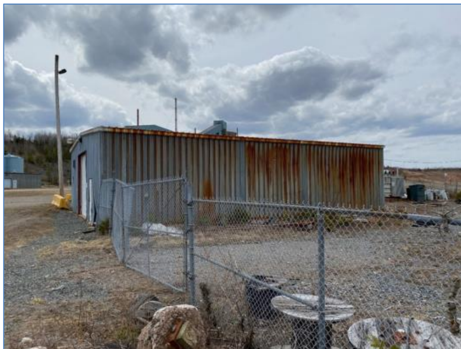
Figure 18-51: Cold Warehouse and Storage Yard
