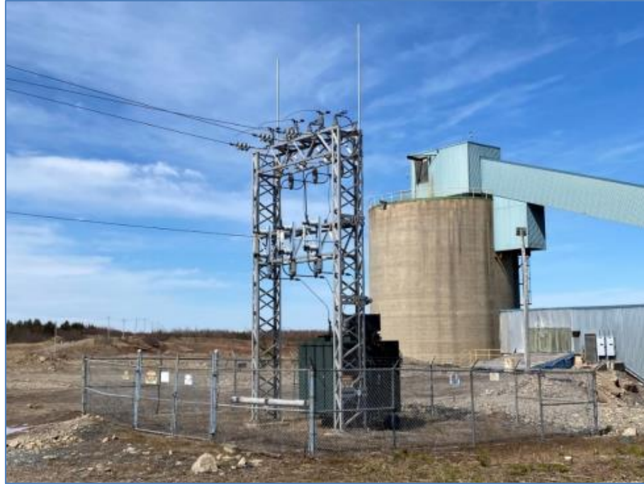
Figure 18-4: 8,000 kVA Transformer
