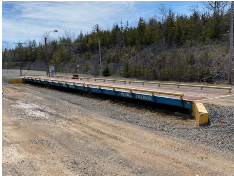
Figure 18-73: Onsite Container Weighbridge
