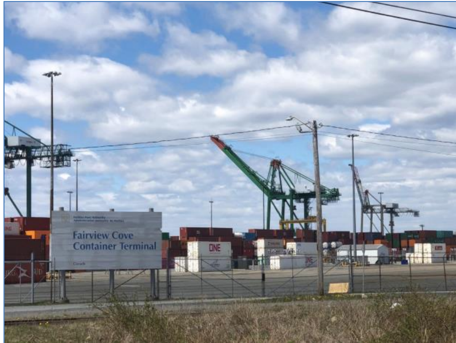
Figure 18-75: Fairview Cove Container Terminal
