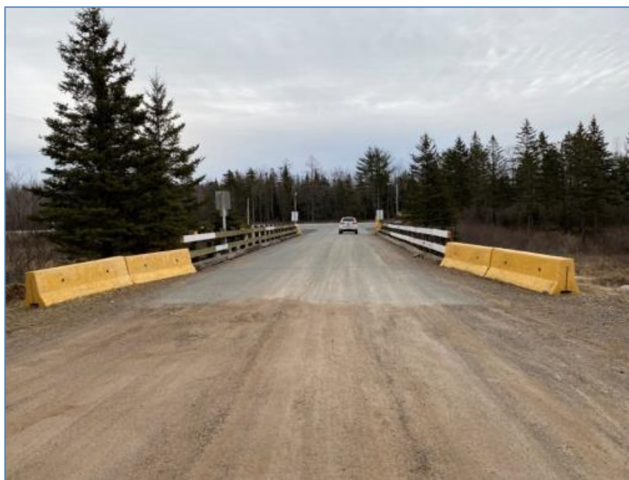
Figure 18-71: ScoZinc's Bridge & Highway Access
