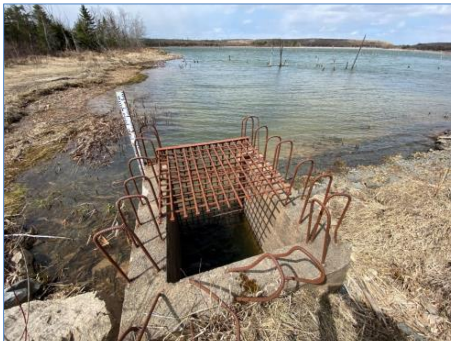
Figure 18-48: Tailings Storage Facility Decant Tower
