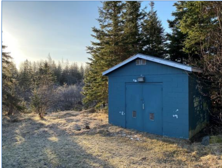
Figure 18-8: Pumping Station at Gay's River
