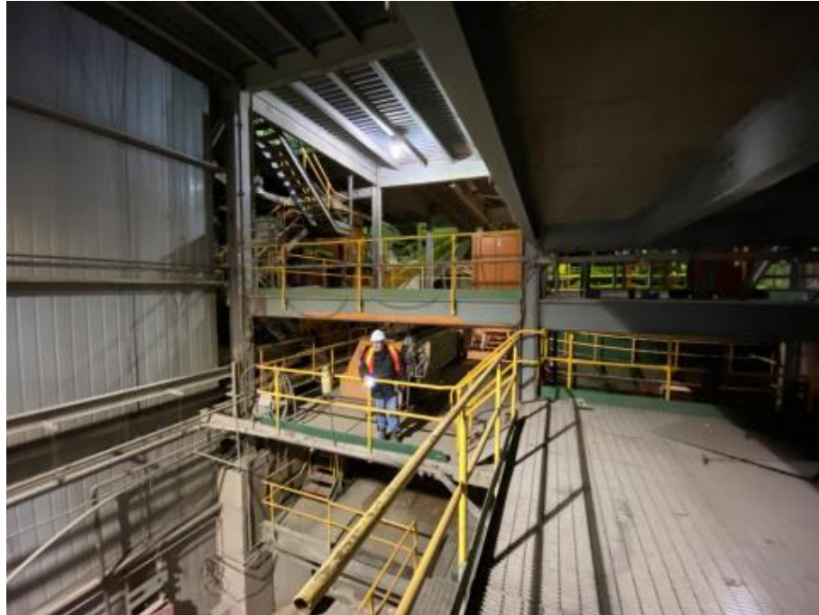
Figure 18-39: Concentrate Dewatering Area
