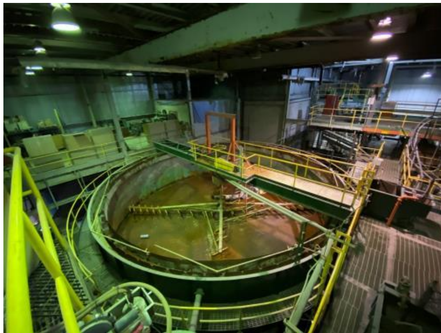
Figure 18-38: Zinc Thickener Tank
