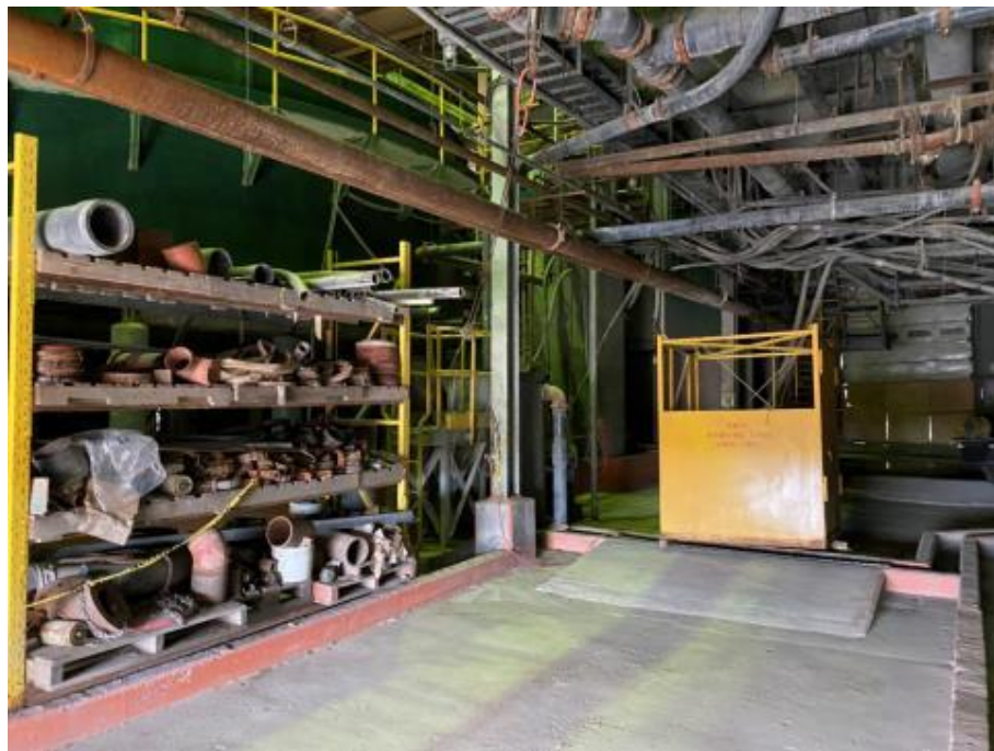
Figure 18-46: Large Ground Floor Maintenance Bays
