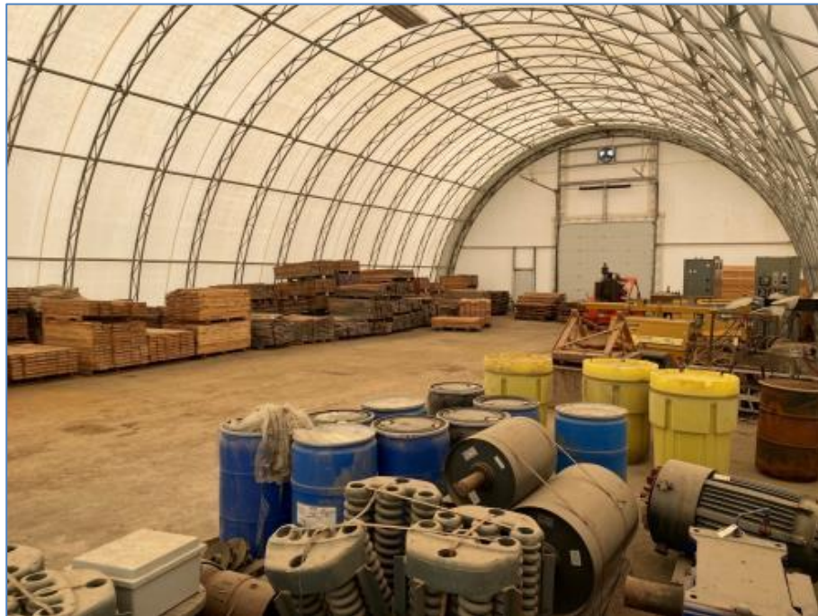
Figure 18-29: Core Storage Building (interior)
