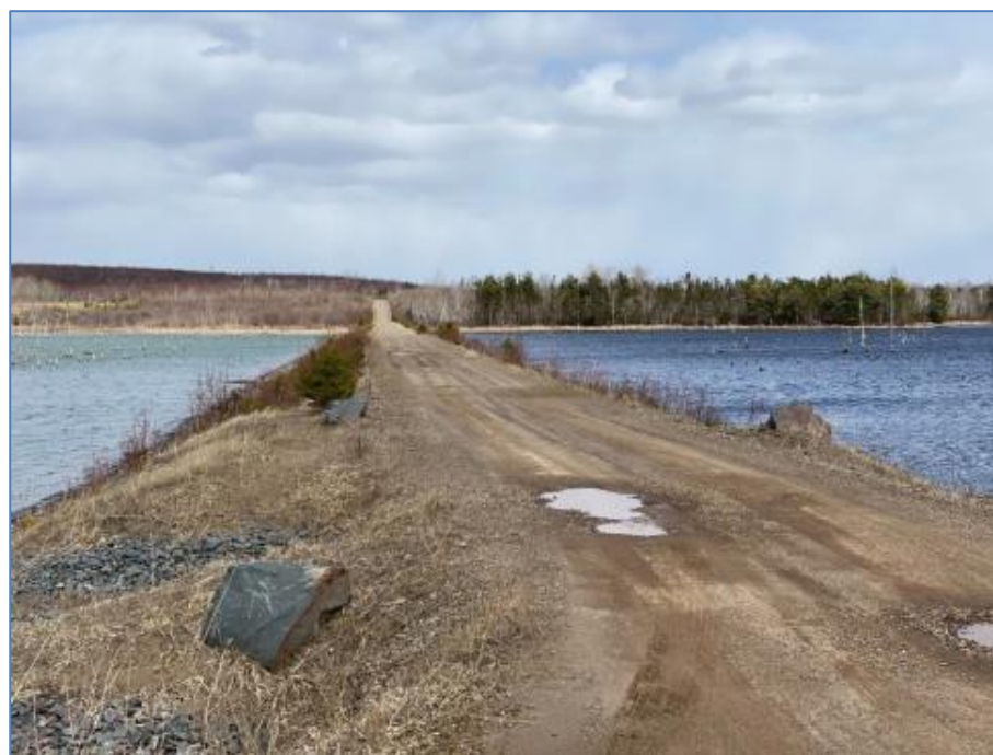
Figure 18-49: Tailings Storage Facility Causeway
