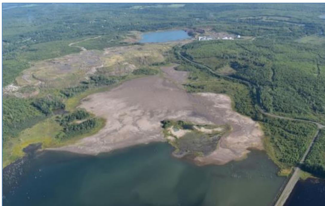
Figure 18-56: Tailings Storage Pond
