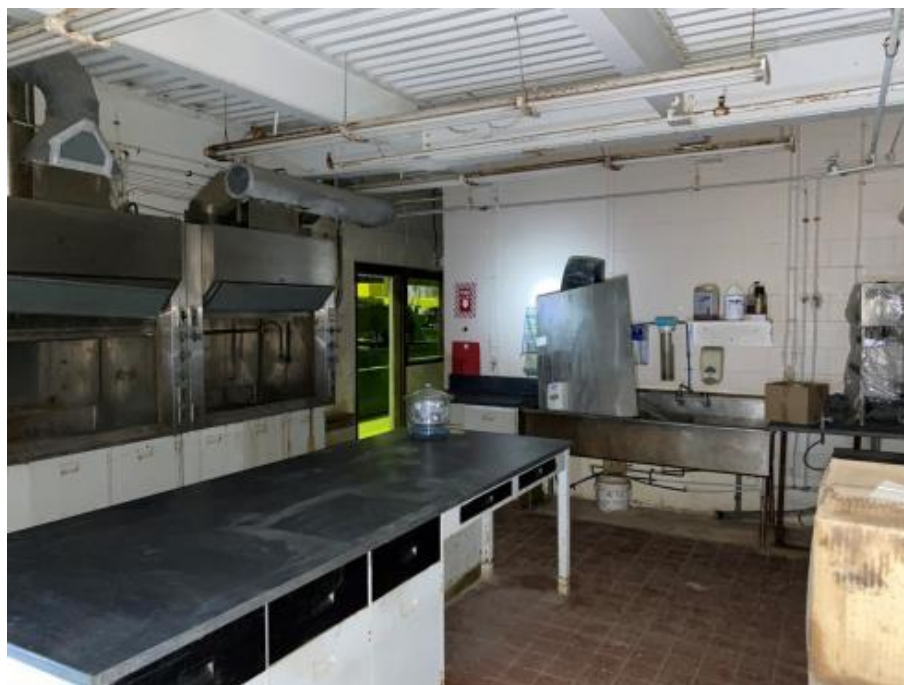
Figure 18-43: Wet Metallurgical Laboratory
