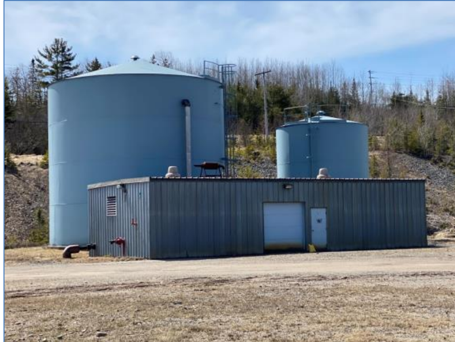
Figure 18-7: Water Treatment Plant and Water Storage
