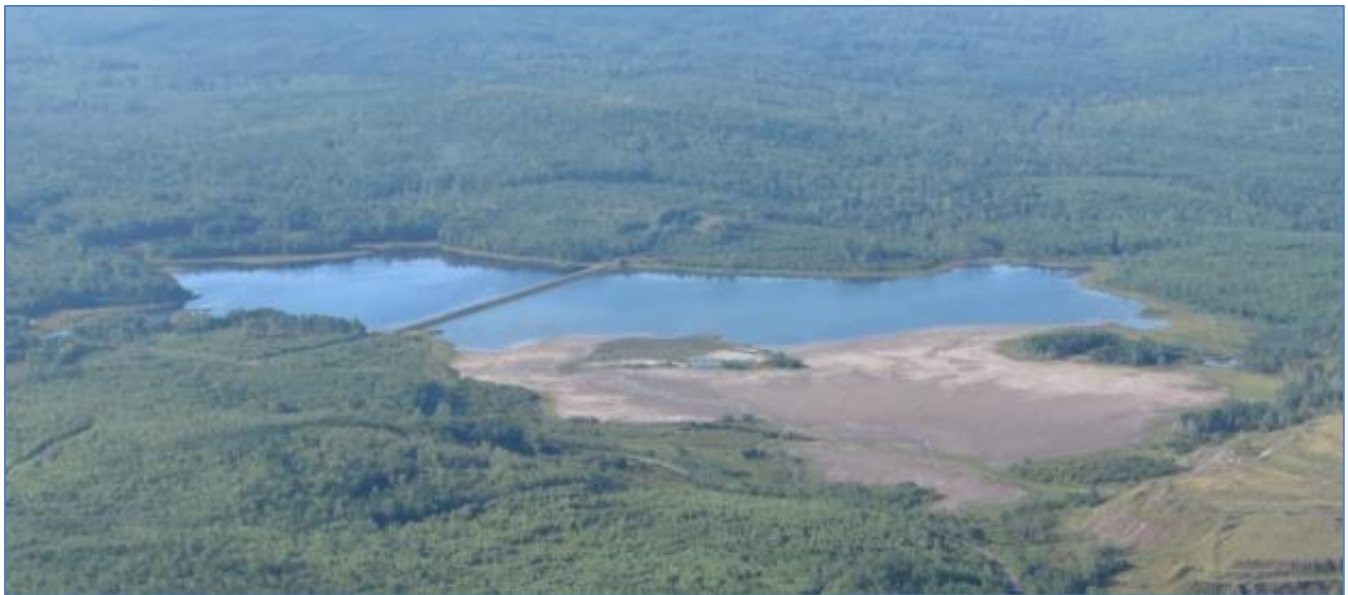
Figure 18-47: Tailings Storage Facility
