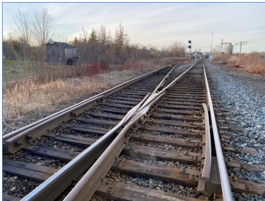
Figure 18-76: Nearby Milford Railway Siding
