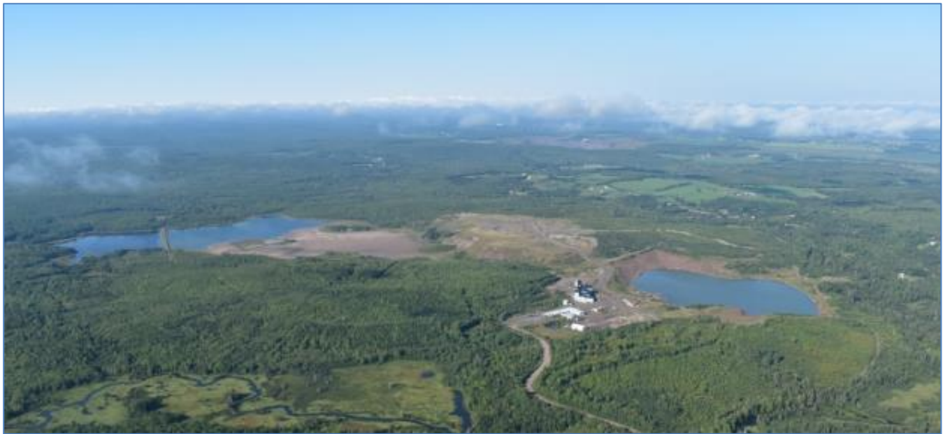
Figure 18-1: Site Aerial Photo (2017)
