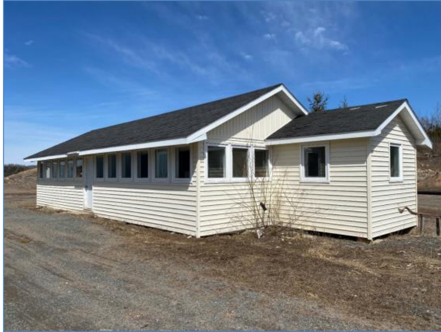
Figure 18-27: Core Preparation Building
