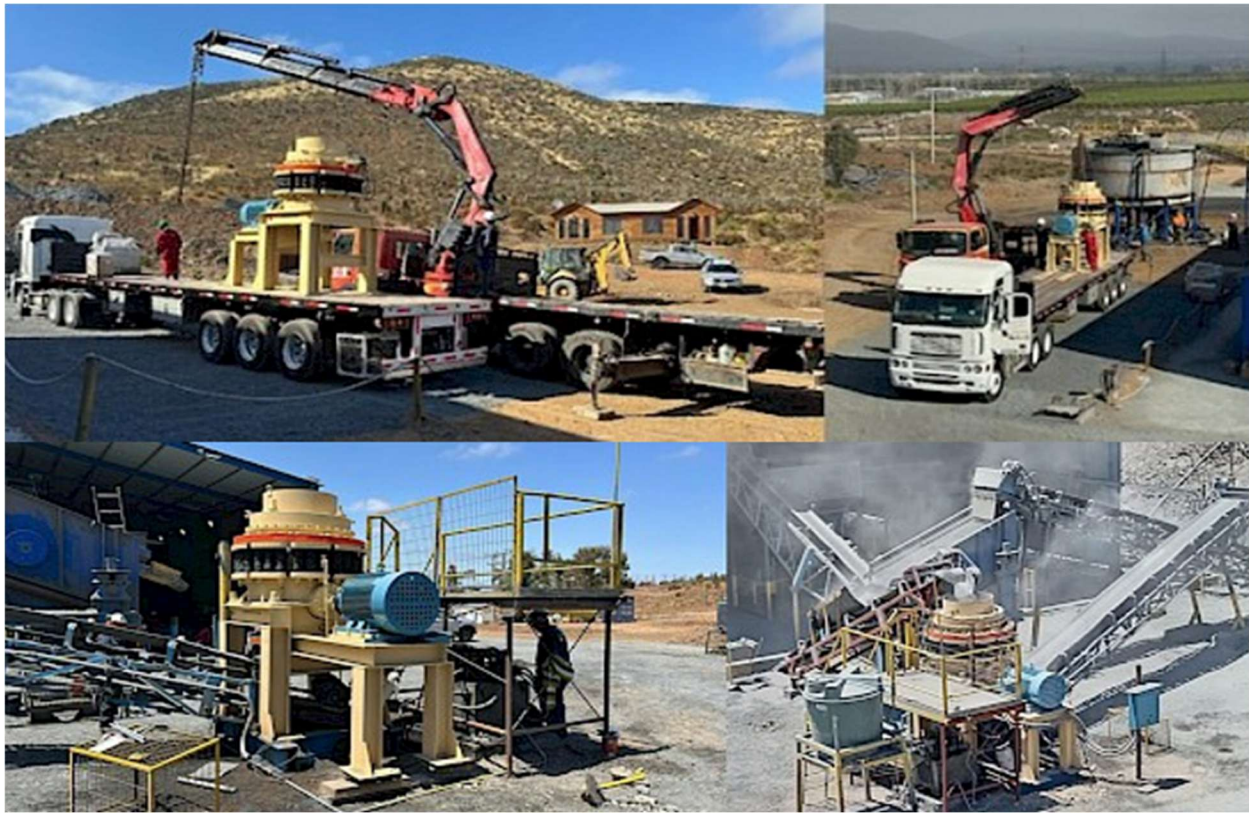
Figure 5. Delivery and Installation of the Cone Crusher
