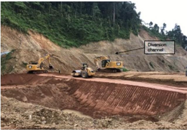
Upstream wall of the cofferdam. (CNW Group/TVI Pacific Inc.)
