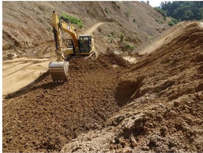
Excavator scarifying the Cofferdam surface prior to compaction. The surface was sealed with a smooth drum compactor due to impending rainfall.
