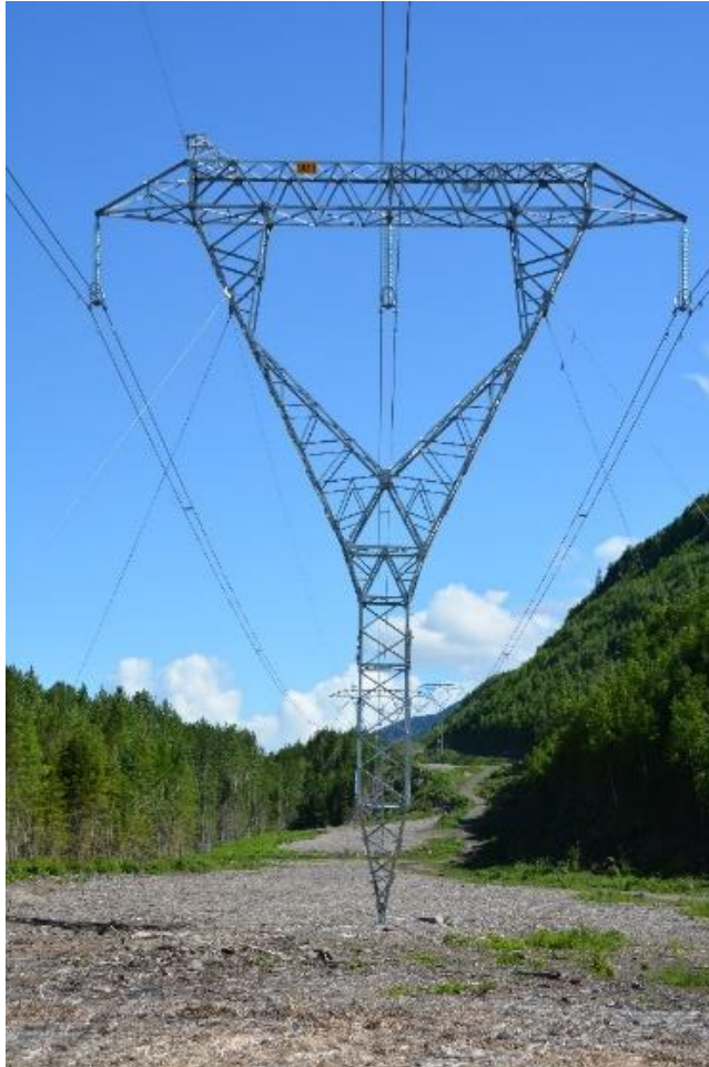
Figure 18-24: Typical 287 kV Guyed Tower
