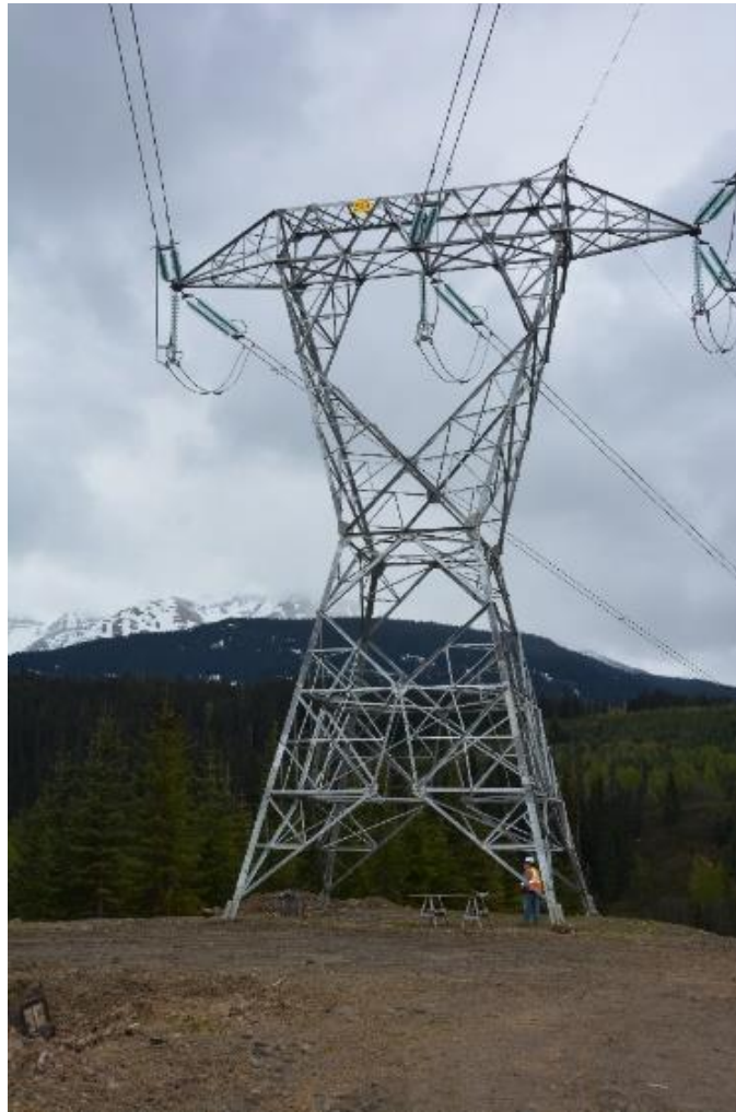
Figure 18-25: Typical 287 kV Self-Supporting Tower
