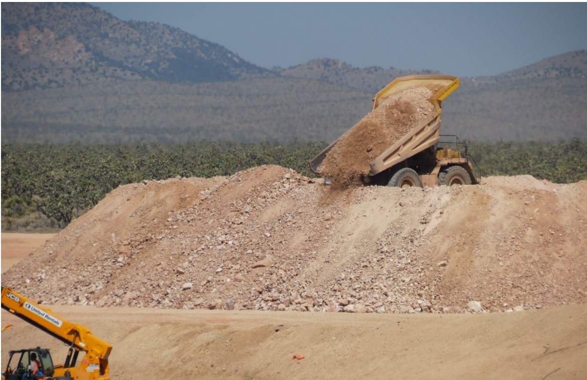
Figure 3 - Stacking ore on leach pad
