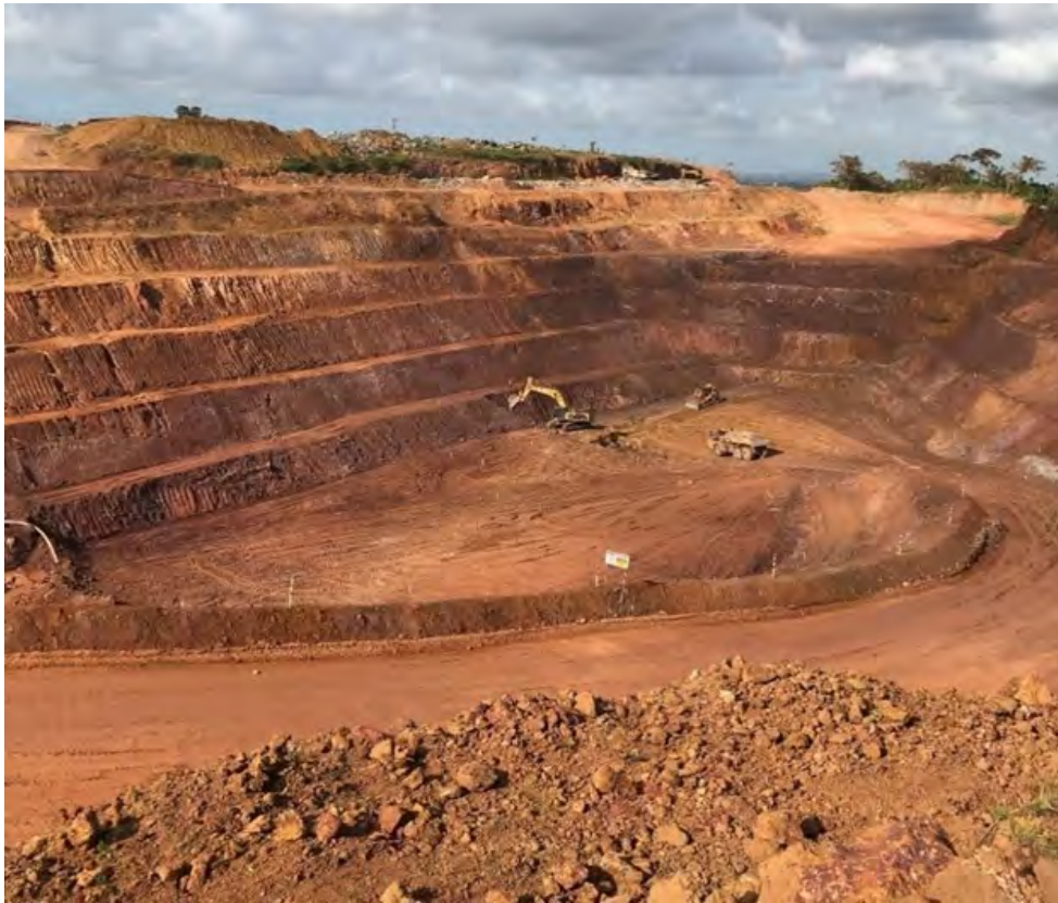
Figure 16-4: Piaba East Wall – August 2021 (Looking West)
