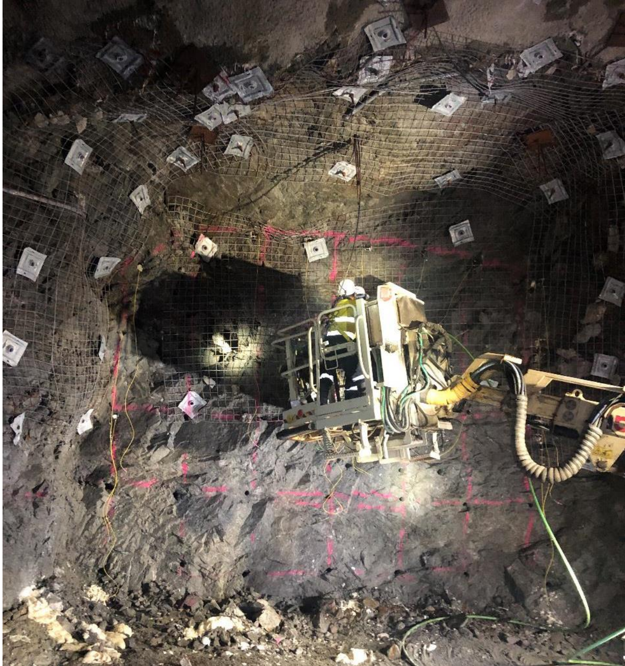
Figure 1 – First Underground Cut at Didipio
