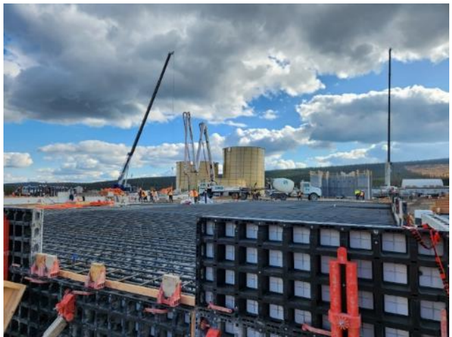
Reagents building civil works – September
