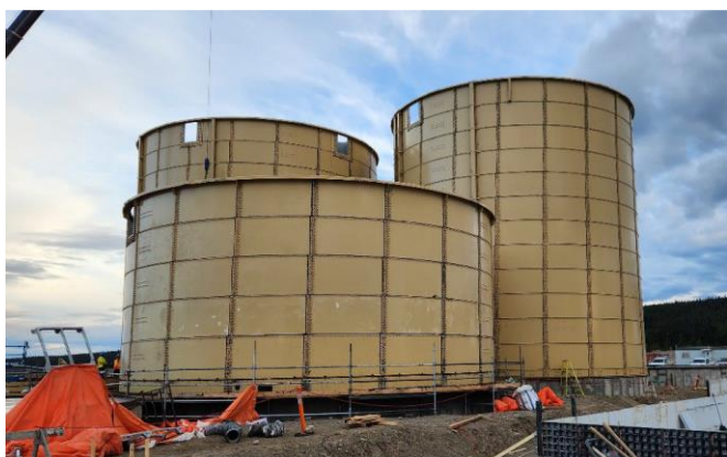
CIL tank construction – October
