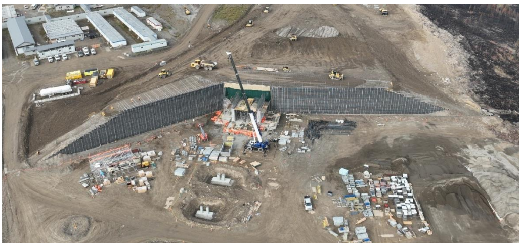
MSE retaining wall/crusher structure and conveyor footings – September
