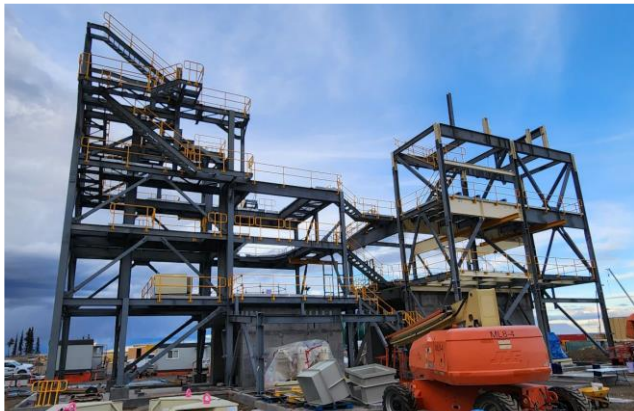
Secondary and tertiary crusher structural steel – October
