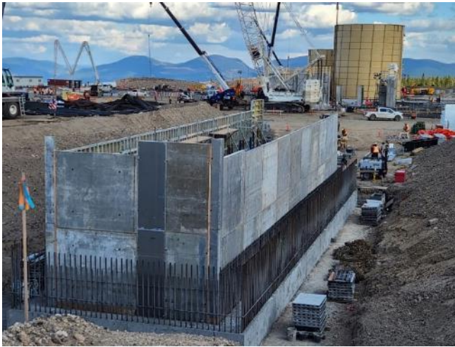
Reclaim tunnel – civil works – September
