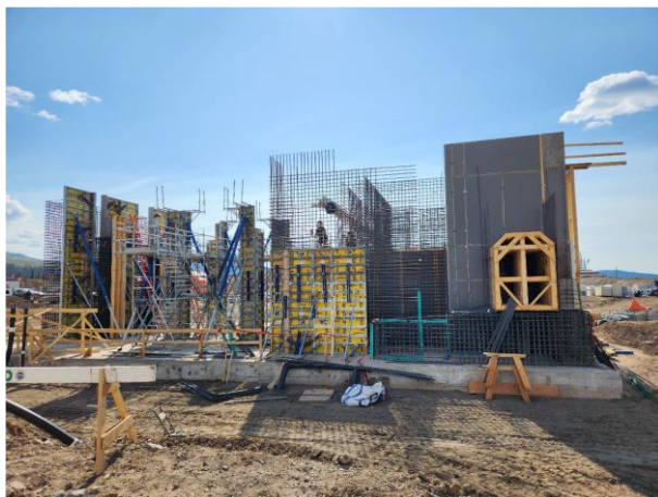
Ball mill foundation and pedestals – June 2023
