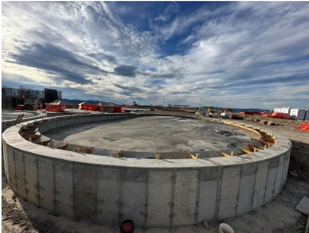
CIL tank foundations – June 2023
