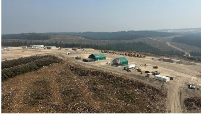
Mobile equipment service area – June 2023
