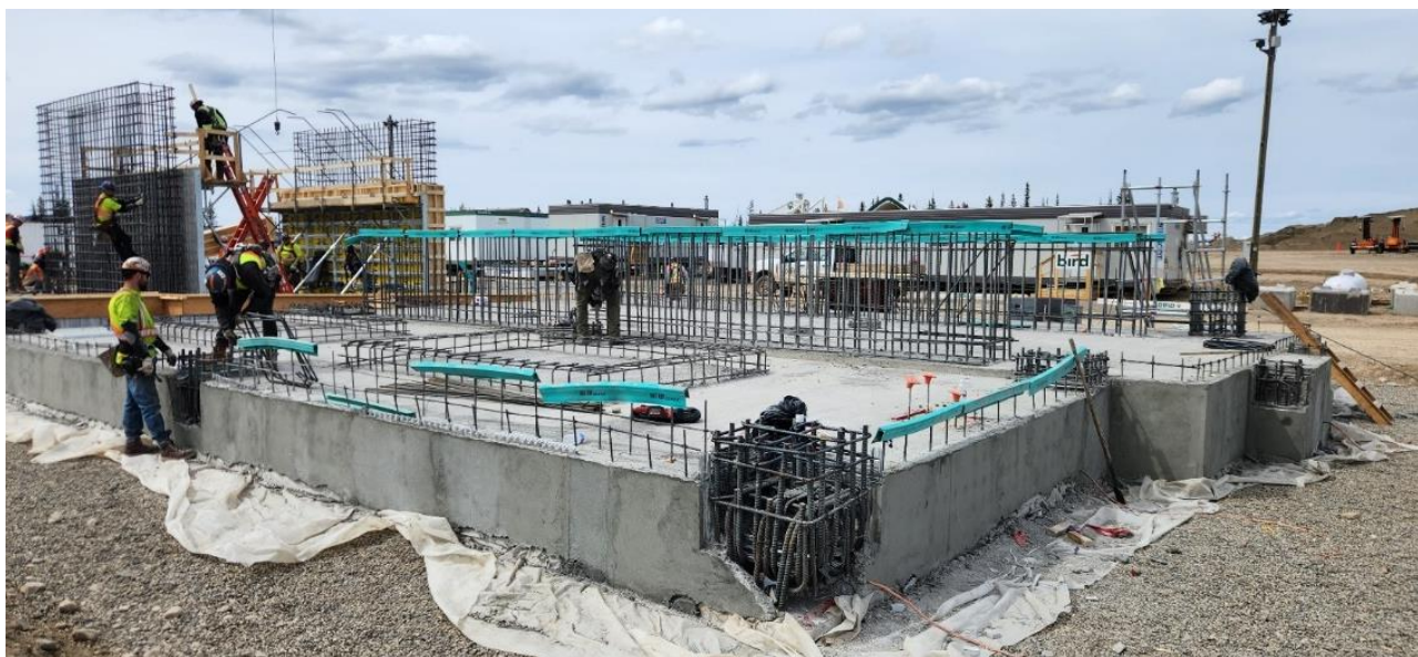
Secondary and tertiary crusher slabs with rebar work underway – June 2023
