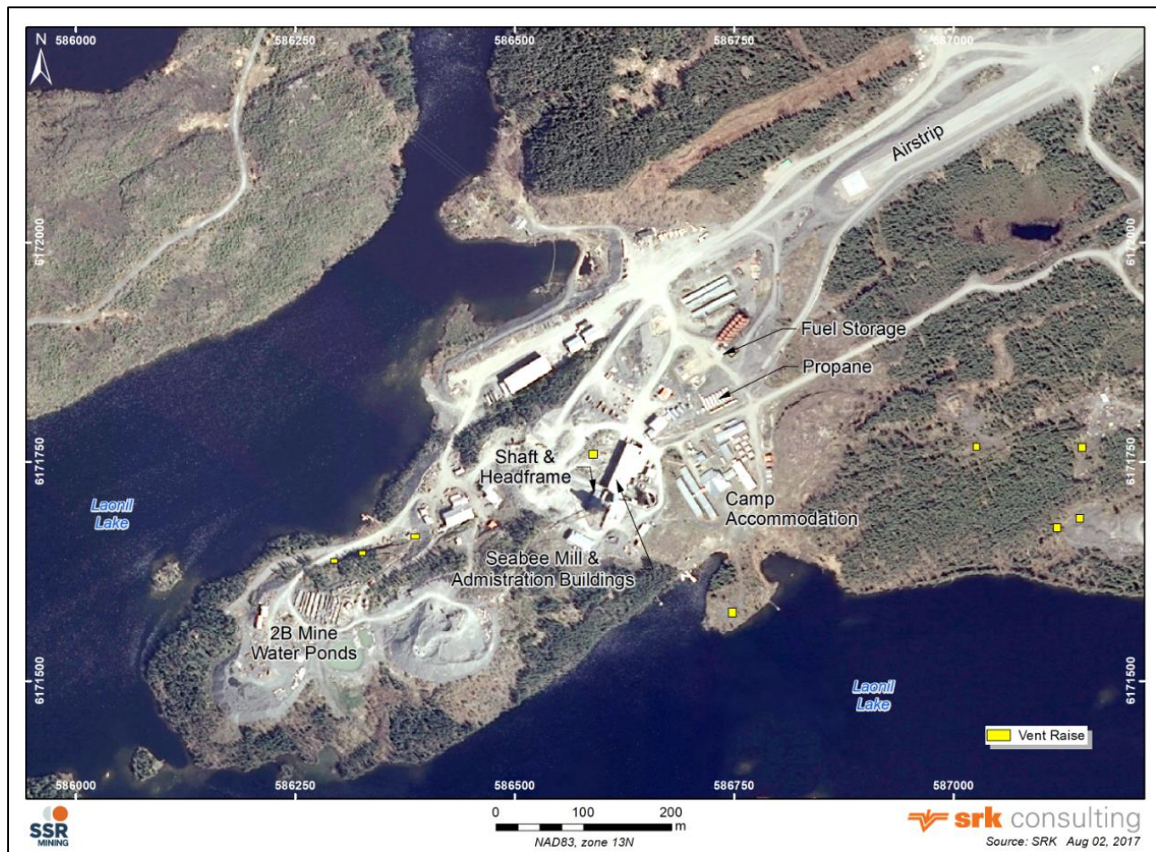
Figure 19: Seabee Mine (Mill Site Infrastructure)
