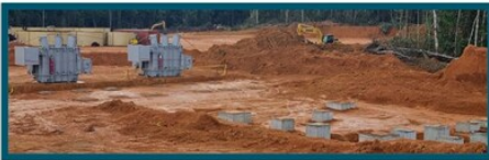
Figure 10 – Site Main Substation Progress (CNW Group/G Mining Ventures Corp)
