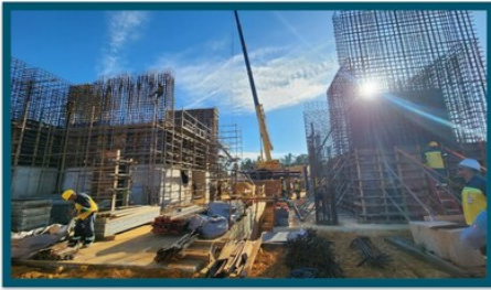
Figure 6 – Mill Foundation and Monument Installation (CNW Group/G Mining Ventures Corp)
