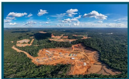
Figure 5 – TZ Site Construction Overview (CNW Group/G Mining Ventures Corp)
