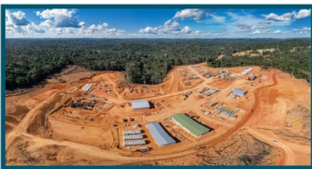
Figure 1 – Mine Infrastructure Area and Process Plant Progress (CNW Group/G Mining Ventures Corp)
