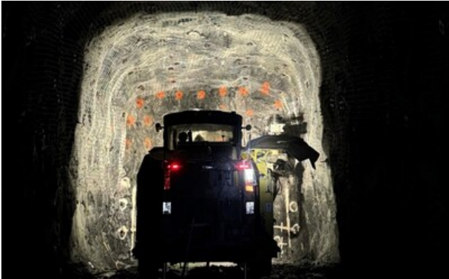
Jumbo Drilling in 120m Level (CNW Group/Foran Mining Corporation)
