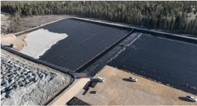
Waste Rock and Ore Pad Liner Installation (CNW Group/Foran Mining Corporation)
