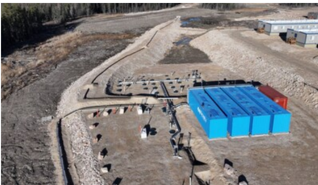
Sewage Treatment Plant and Septic Field (CNW Group/Foran Mining Corporation)
