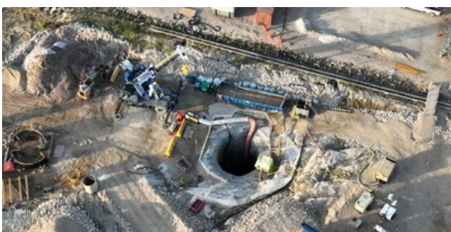
Fresh Air Raise (CNW Group/Foran Mining Corporation)
