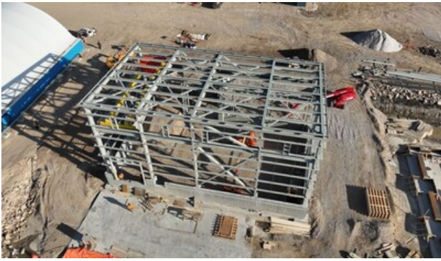
Steel Erection at Surface Maintenance Shop (CNW Group/Foran Mining Corporation)
