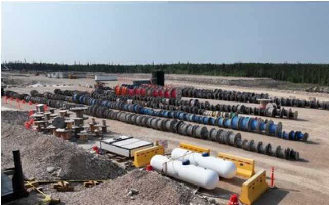
Electrical Cable Reel Storage (CNW Group/Foran Mining Corporation)
