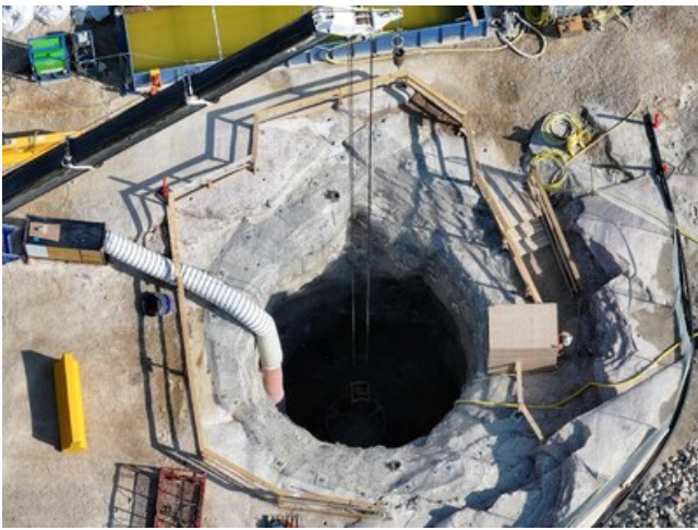
Main Surface Fresh Air Raise Collar Sinking (CNW Group/Foran Mining Corporation)
