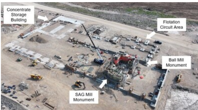
Processing Plant Form and Concrete Works (CNW Group/Foran Mining Corporation)
