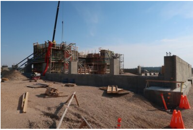
Grinding Area Concrete Works (CNW Group/Foran Mining Corporation)
