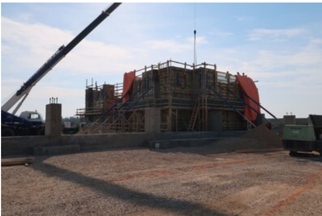
Mill Monument Construction (CNW Group/Foran Mining Corporation)
