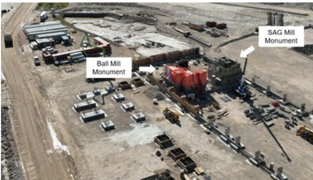
Processing Plant Form and Concrete Work (CNW Group/Foran Mining Corporation)
