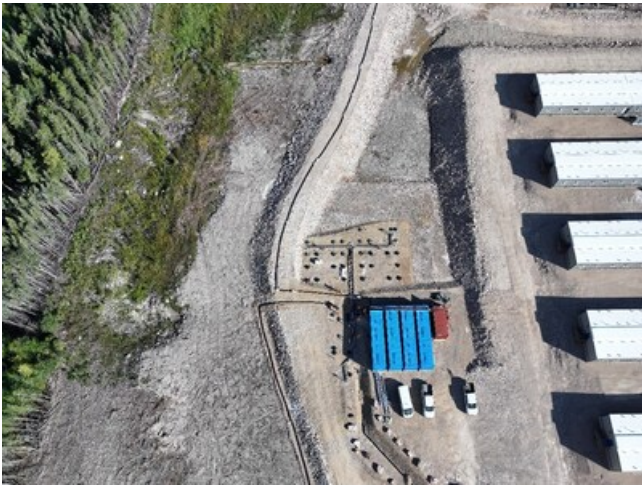
Site Septic (CNW Group/Foran Mining Corporation)
