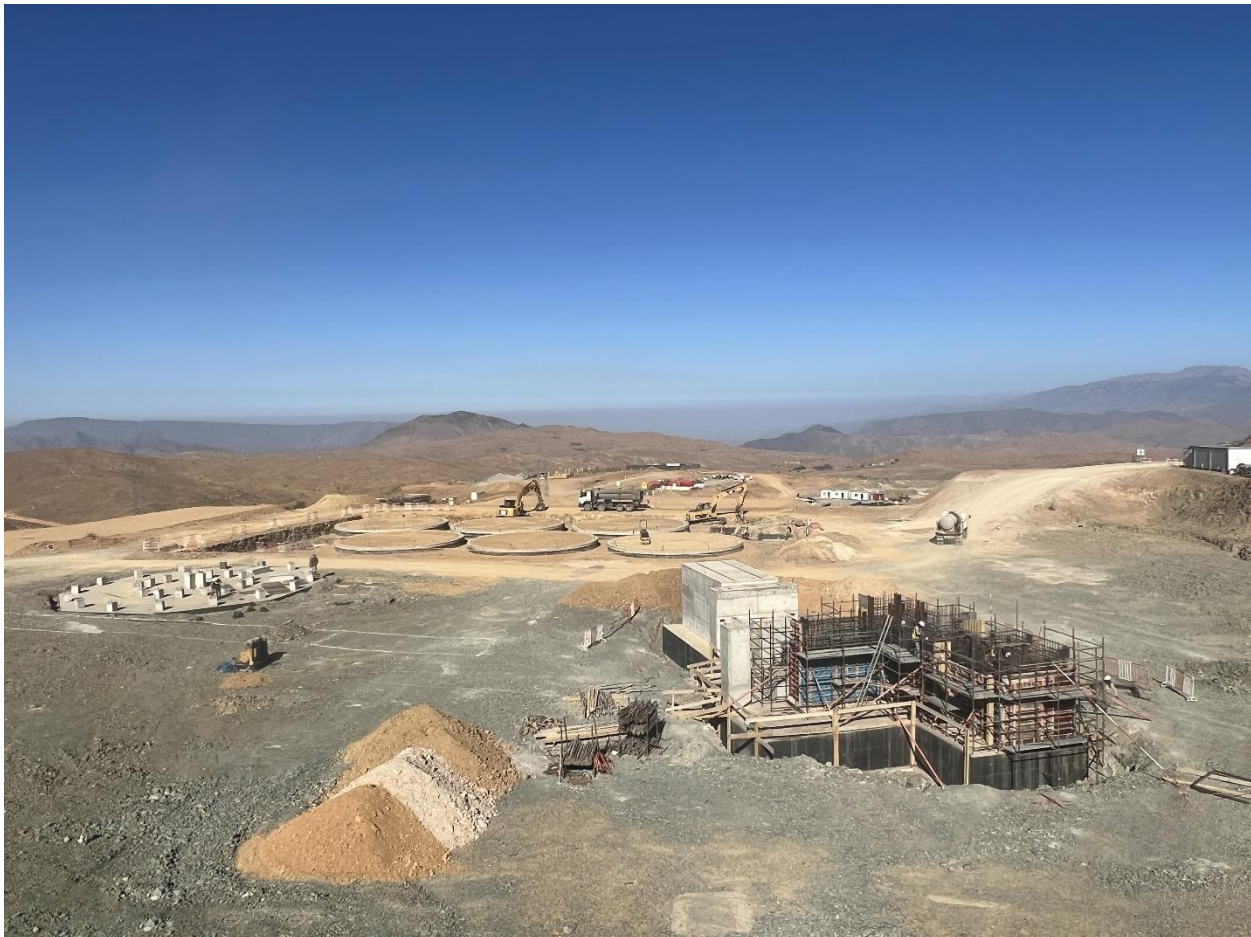
Figure 1 – Ongoing civil and concrete work at the new Zgounder processing plant
