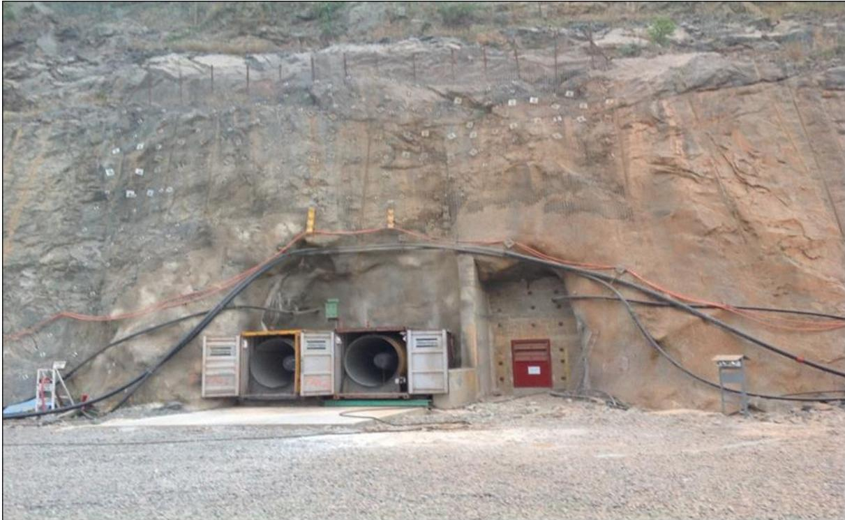
Figure 16-18: Akoti 2x315kw Exhaust Swedvent Fans
