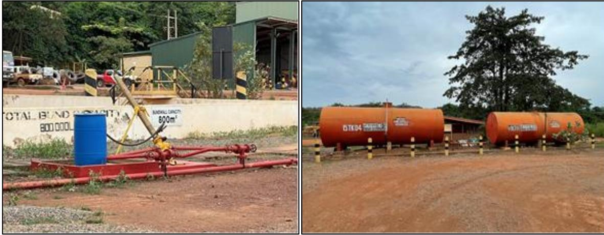
**Figure 18-13: Fire Suppression System at Mine Service Area Fuel Farm**
