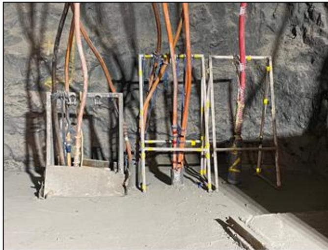
*Figure 18-19: HV Cables through Service Holes at Suraw*
